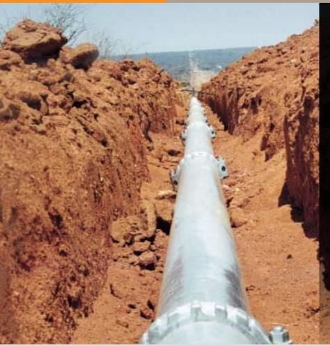
The Klambon piping system is widely recognised as the most efficient pipe joining system available. The shouldered and grooved systems include piping, couplings and a comprehensive range of fittings.
